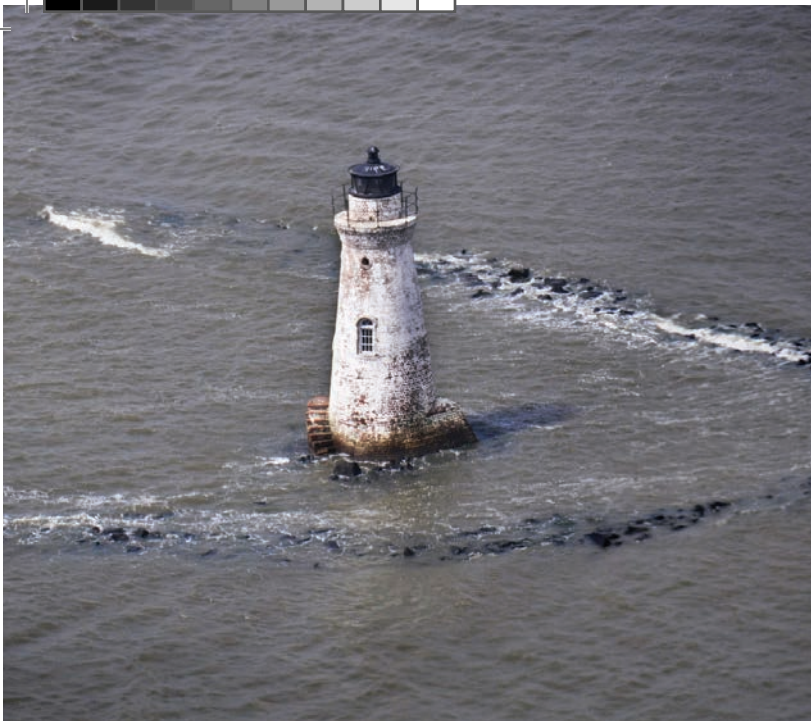
During high tide, the base of Cockspar Lighthouse is awash with the Savannah River.
