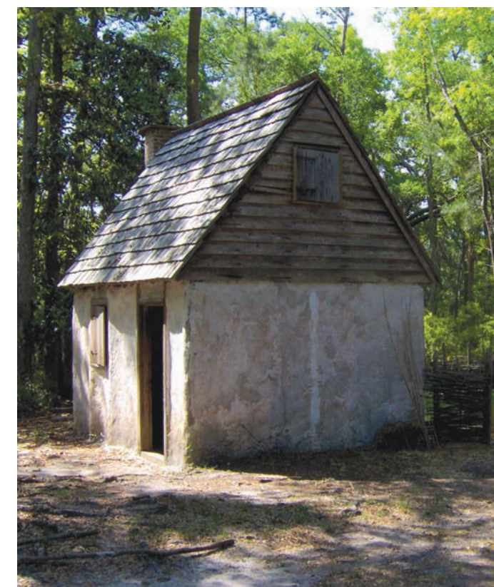
A replica of a Colonial-era wattle-and-daub hut, which usually housed enslaved people.
